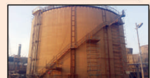
Ammonia Tank maintenance
